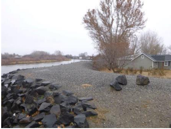
Photo 1. Levee south of bridge, facing south
