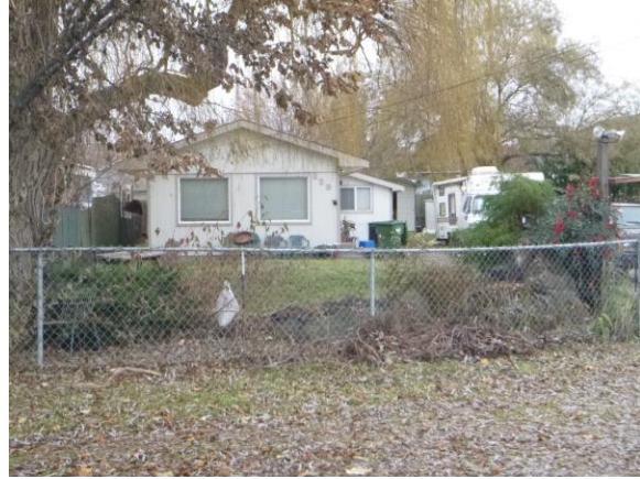
Viewing southwest Northeast oblique 2014
