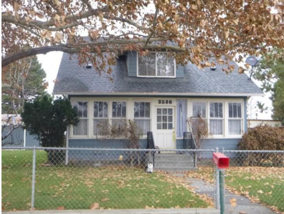
Viewing north South facade 2014
