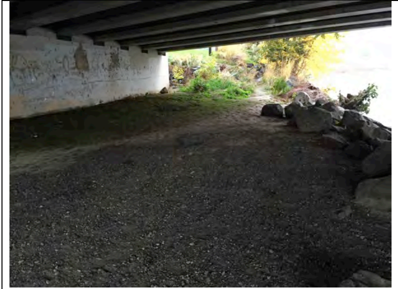
Under west side of bridge facing north
