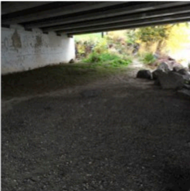
Under Bridge Facing North
