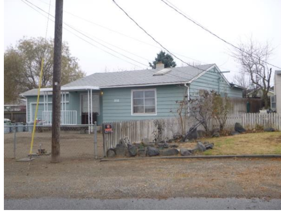
Viewing southwest Northeast oblique 2014
