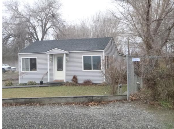
Viewing southwest Northeast oblique 2014
