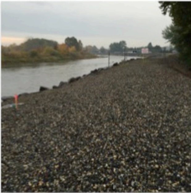
Levee South of Van Giesen Bridge-facing south
