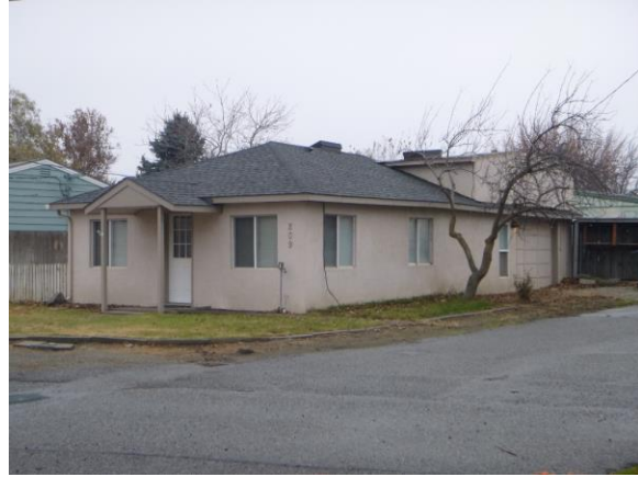
Viewing southwest Northeast oblique 2014
