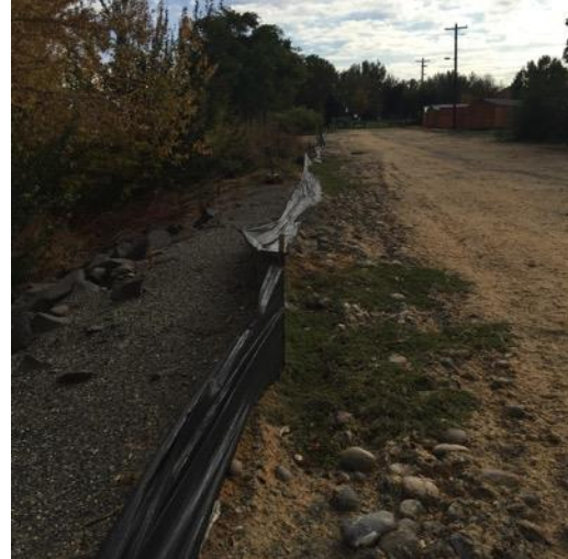
Photo 3. Gravel roadway north of bridge, facing south.
