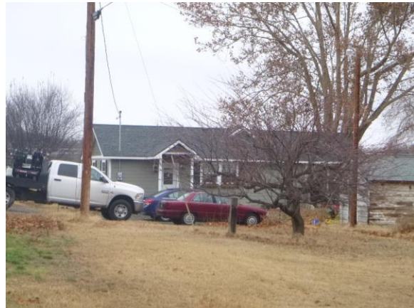
Viewing north South face 2014
