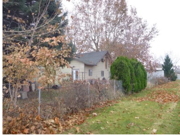
Viewing southwest Northeast oblique 2014
