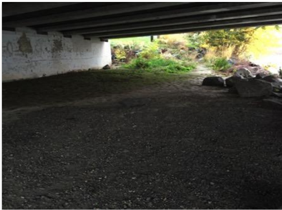
Photo 2. Underside of bridge, facing north
