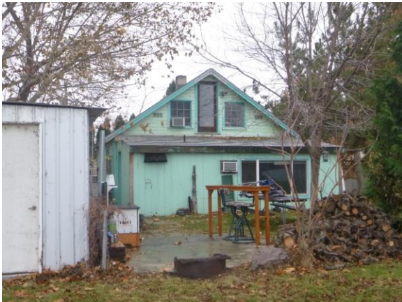
Viewing southwest Northeast oblique 2014
